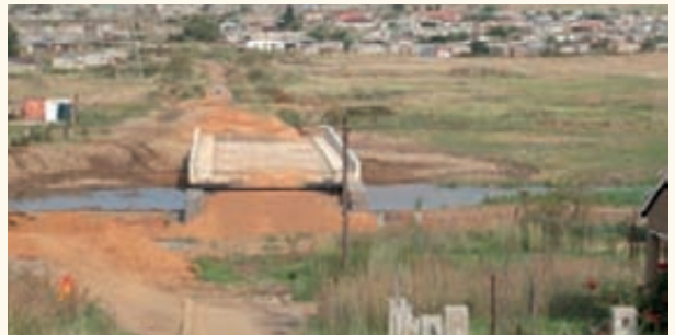
Bhanya River Bridge after construction
