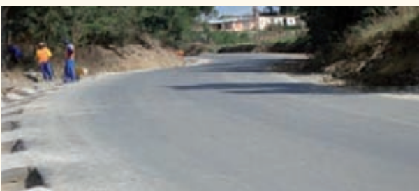
Section of D877 during Construction
