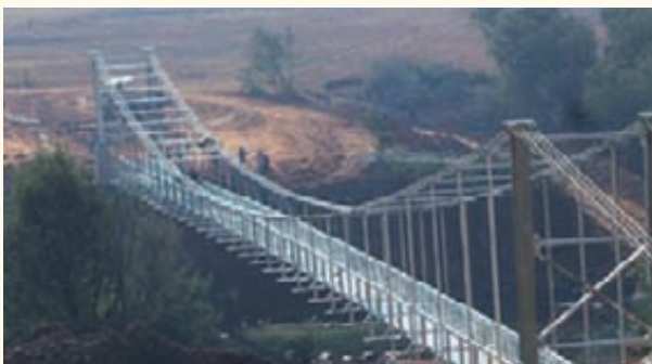
Lotheni Pedestrian Bridge after construction
