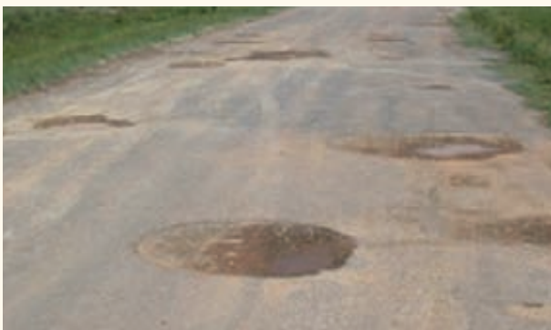
Road P28/1 before resealing
