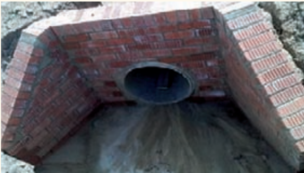
Ntalantala headwall after construction
