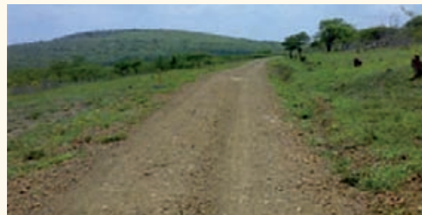
Local Road A2162 after Construction
