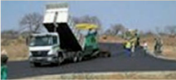
Section of P218/P710 during Construction
