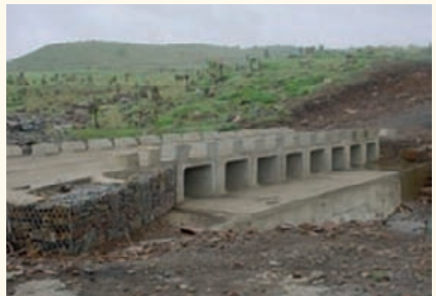
Mkhumbane Structure after Construction
