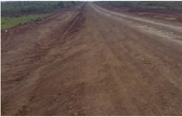
P348 after Construction
