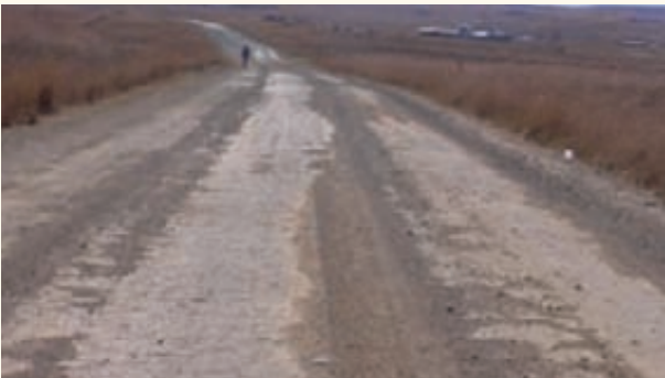
P 361 before construction
