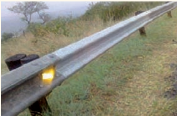
Guardrail repairs after repair
