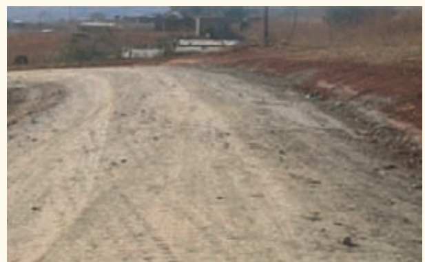
Amabomvu Road after Construction
