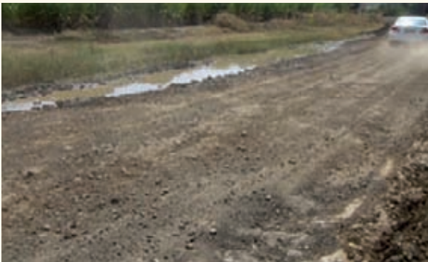
P518 - Headwall before installations
