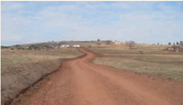
Cengeni Local Road after Construction
