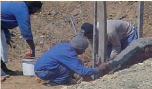
Ntalantala headwall before construction
