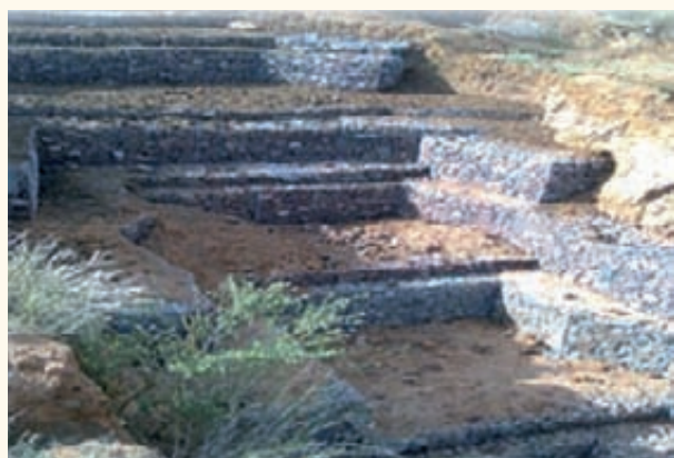
A1223 after gabion repairs and installation
