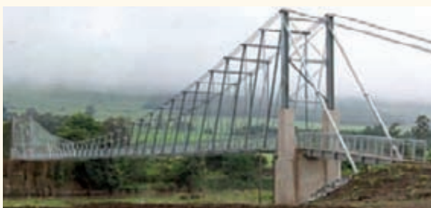
Mzimkhulu Structure after construction
