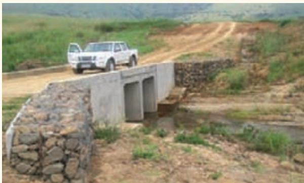
Isibabe Causeway after construction
