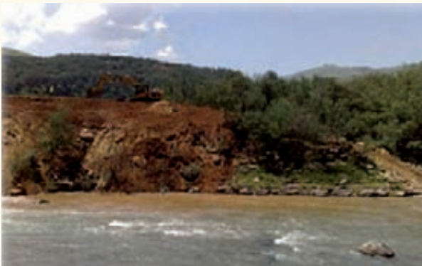
Lotheni Pedestrian Bridge before construction
