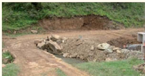
Road L1331 after construction
