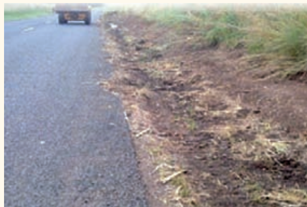
Subsoil drainage on P6/1
