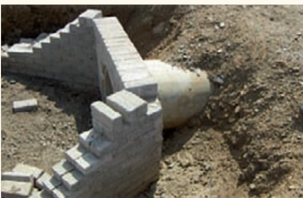
P518 - Headwall after installations
