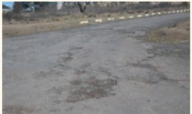
P154 before after resealing
