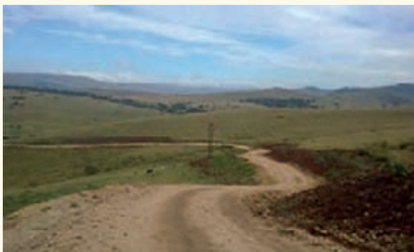
Kweyezulu Local Road After Construction
