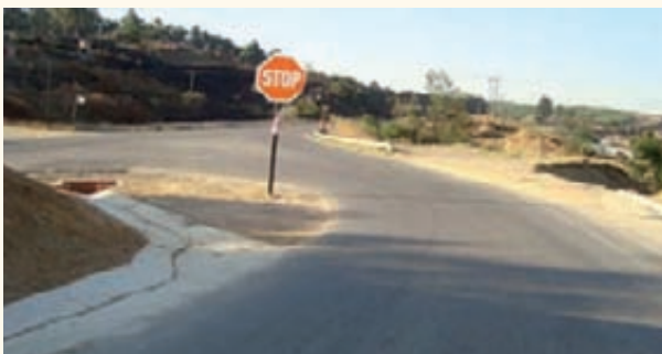
Completed section of P487
