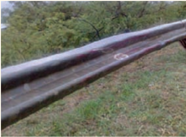
Guardrail repairs before repair
