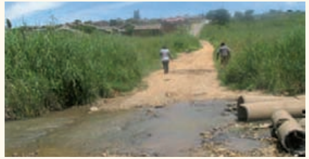
Bhanya River Bridge before construction
