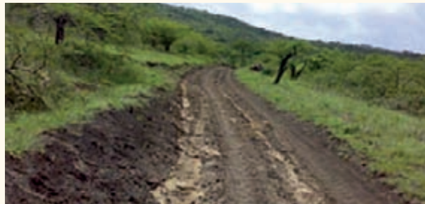
Local Road A2162 before Construction
