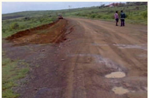
P348 before Construction
