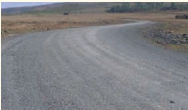
P 361 before construction
