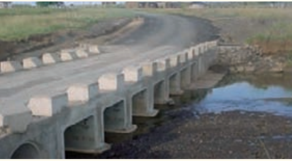
A2105 Structure after construction
