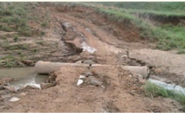
Isibabe Causeway before construction
