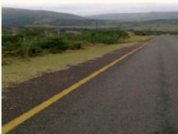
After Drain Clearing and Verge Maintenance
