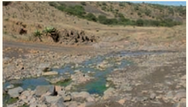
Mkhumbane Structure before Construction
