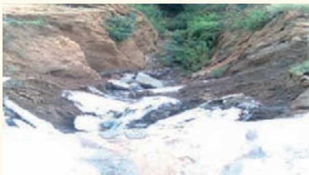
A1223 before gabion repairs and installation
