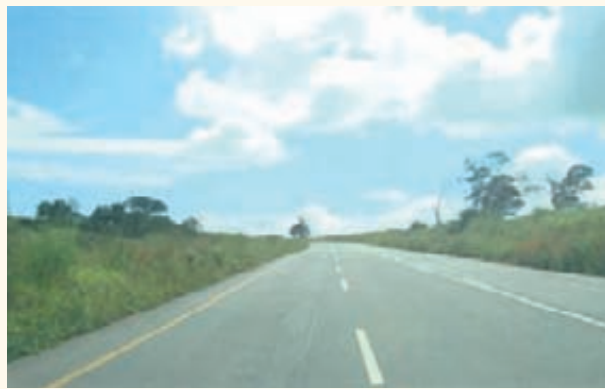
P5/2 After Rehabilitation
