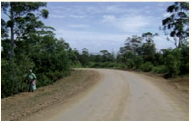
District Road D2414 after blading
